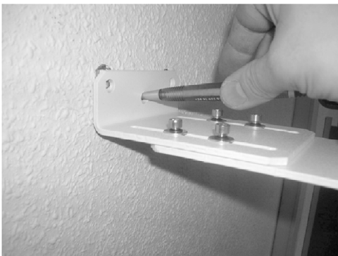
Illustration 3-14 Bracket Fixations Drilling
