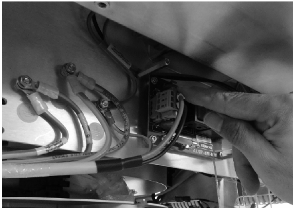
Illustration 6-12 Input Module Connection
